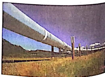
The Trans-Alaska Pipeline carries crude oil 1,284 kilometres through Alaska. The pipeline is 1.2 metres in diameter and can transport 318 million litres of crude oil a day.
